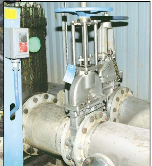
Filter isolation installation.
