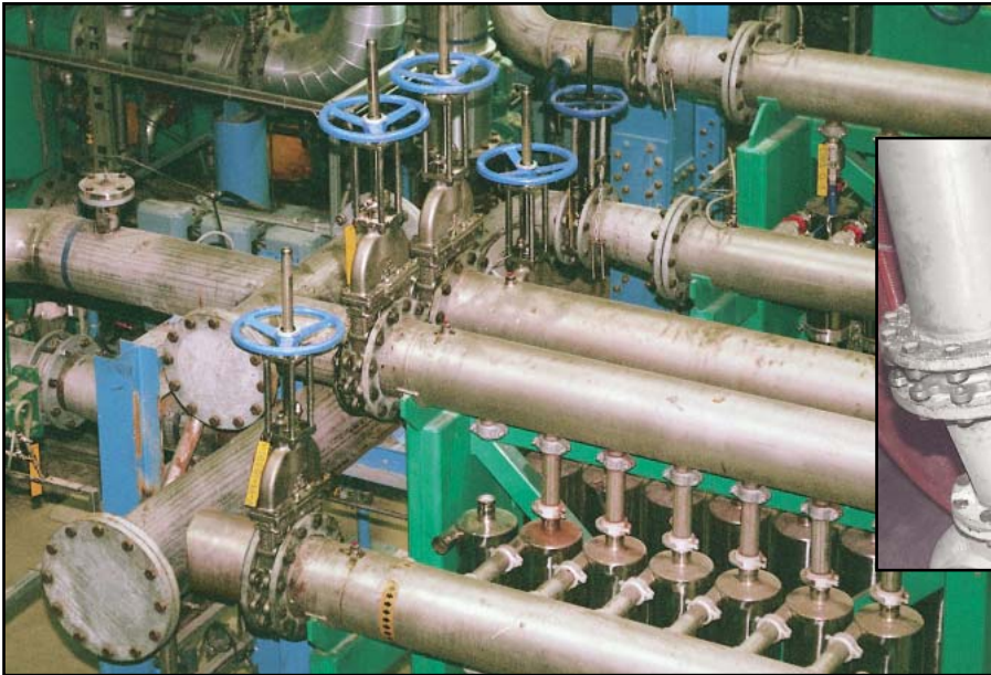
Centrifugal cleaner isolation. Pressure around 25-35 psi (1.7-2.4 bar) 2.5% pulp.
