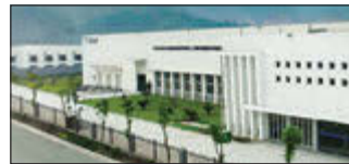
Suzhou, China Velan Valve (Suzhou) Co., Ltd.
