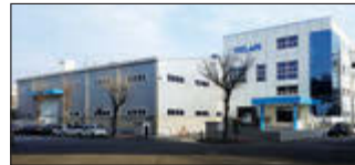
Ansan City, South Korea Velan Ltd., Plant 1
