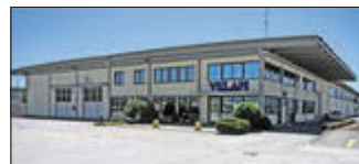
Lucca, Italy Velan ABV S.r.l., Plant 2
