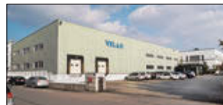
Ansan City, South Korea Velan Ltd., Plant 2
