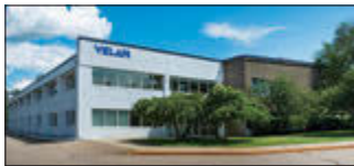
Williston, VT, U.S.A. Velan Valve Corp., Plant 3
