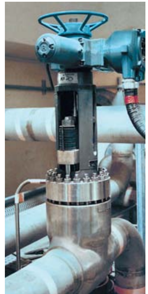
A Velan bolted bonnet gate valve in a PHT transfer system in a CANDU nuclear reactor.
