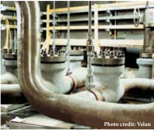
Velan forged bolted bonnet check valves in active nuclear plant drainage.
