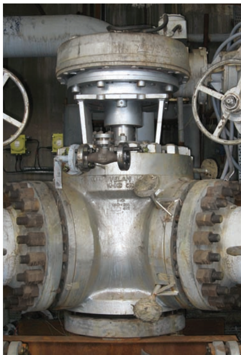
Velan is the only company to date to supply a class 900 16" (400 mm) four-way switch valve to a delayed coker installation.
