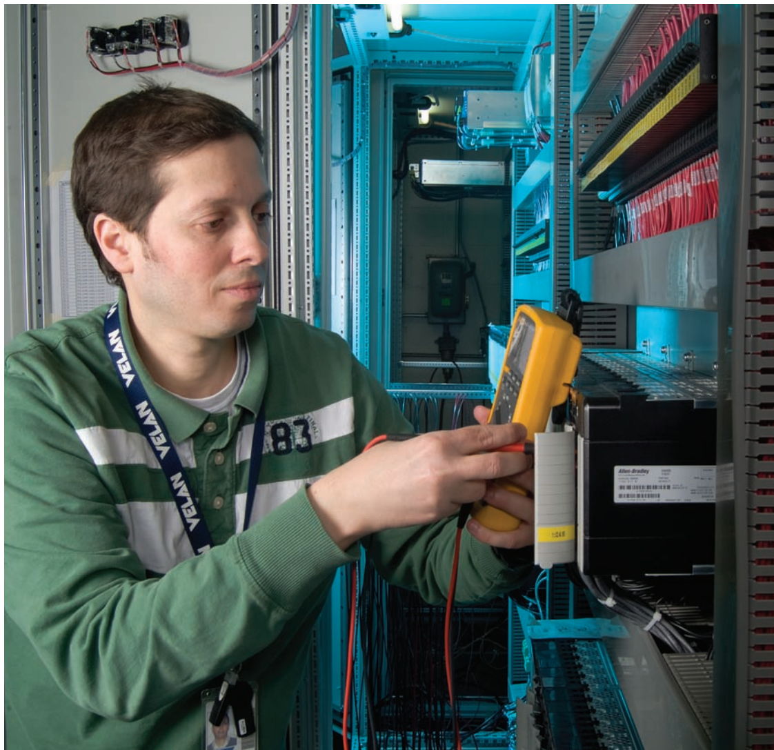
Working behind the scenes, Hicham Guessous Doss, Engineer, Electrical Control Systems, tests the voltage on a PLC (Programmable Logic Controller) input-output module.
