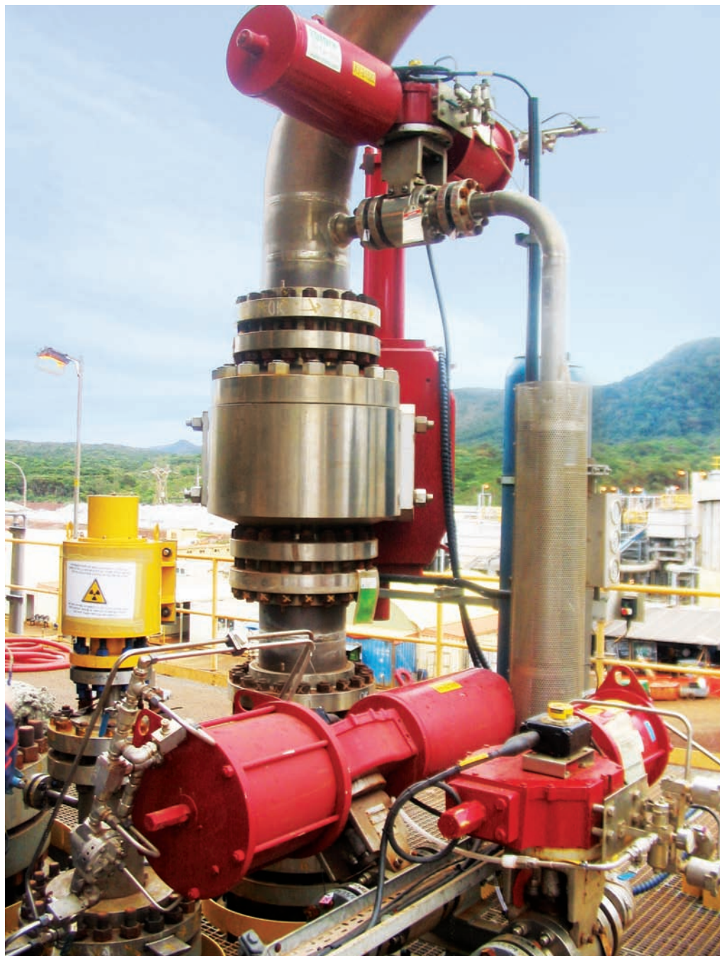
A Velan Type R severe service metal-seated ball valve installation at the Goro project site in New Caledonia.
