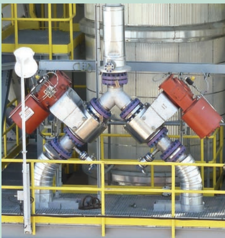
Two 10" Class 150, super duplex, stainless steel Velan Securaseal valves in the feed circuit at a typical HPAL installation.
