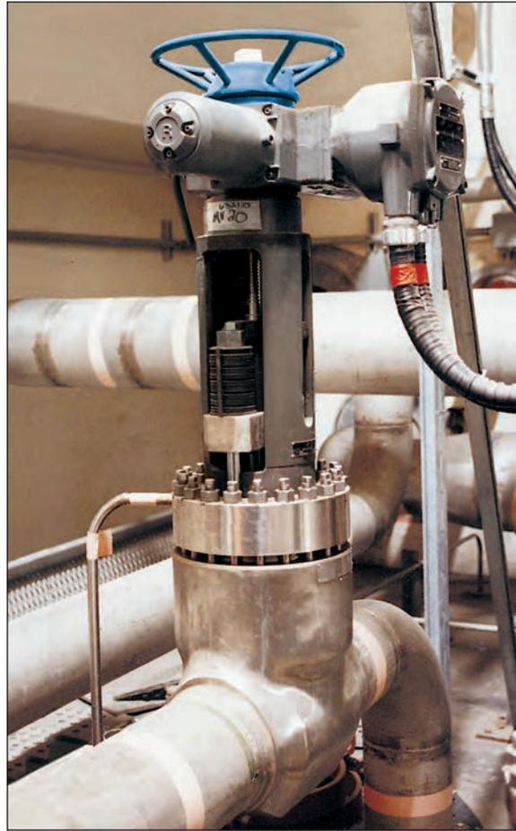
A Velan bolted bonnet valve in a PHT transfer system.
