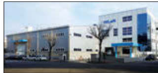
Ansan City, South Korea Velan Ltd., Plant 1
