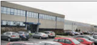
Montreal, Canada Velan Inc., Plant 1
