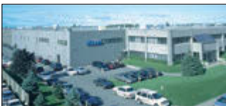
Montreal, Canada Velan Inc., Plant 2 and 7
