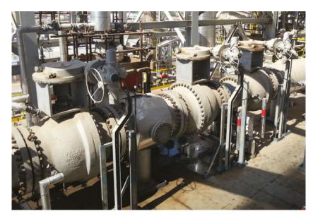
Three 36" Class 300 two-way metal-seated ball valves installed at a refinery in Egypt. Velan's Aftermarket and Technical Services provided on site assistance with the start-up.
