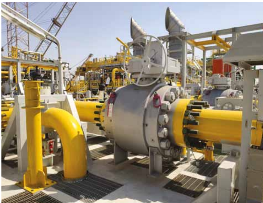
20" Class 2500 three-piece forged bolted body high pressure compact ball valve installed in a FPSO unit in offshore service.
