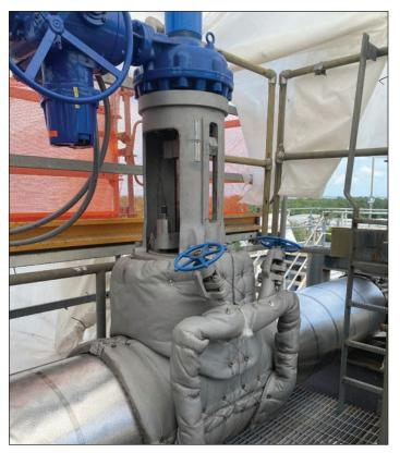
This 14" Class 2500 forged pressure seal valve, installed in a power plant in Florida–part of a large long-term contract with Velan to supply over 100 (12"–24") valves over 5 years.
