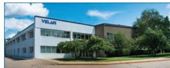
Williston, VT, USA Velan Valve Corp.
