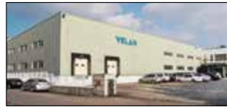
Ansan City, South Korea Velan Ltd., Plant 2
