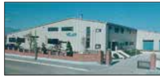
Ansan City, South Korea Velan Ltd., Plant 1
