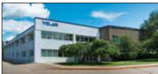
Williston, VT, U.S.A. Velan Valve Corp., Plant 3
