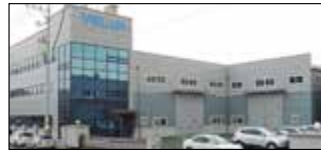
Ansan City, South Korea Velan Ltd., Plant 3
