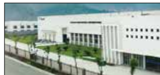
Suzhou, China Velan Valve (Suzhou) Co., Ltd.
